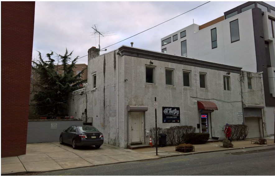
EXISTING BUILDING AT 613-19 S. 24TH ST VIEW SOUTHEAST ON S. 24TH ST
