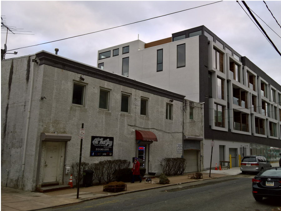
EXISTING BUILDING AT 613-19 S. 24TH ST VIEW SOUTHEAST ON S. 24TH ST
