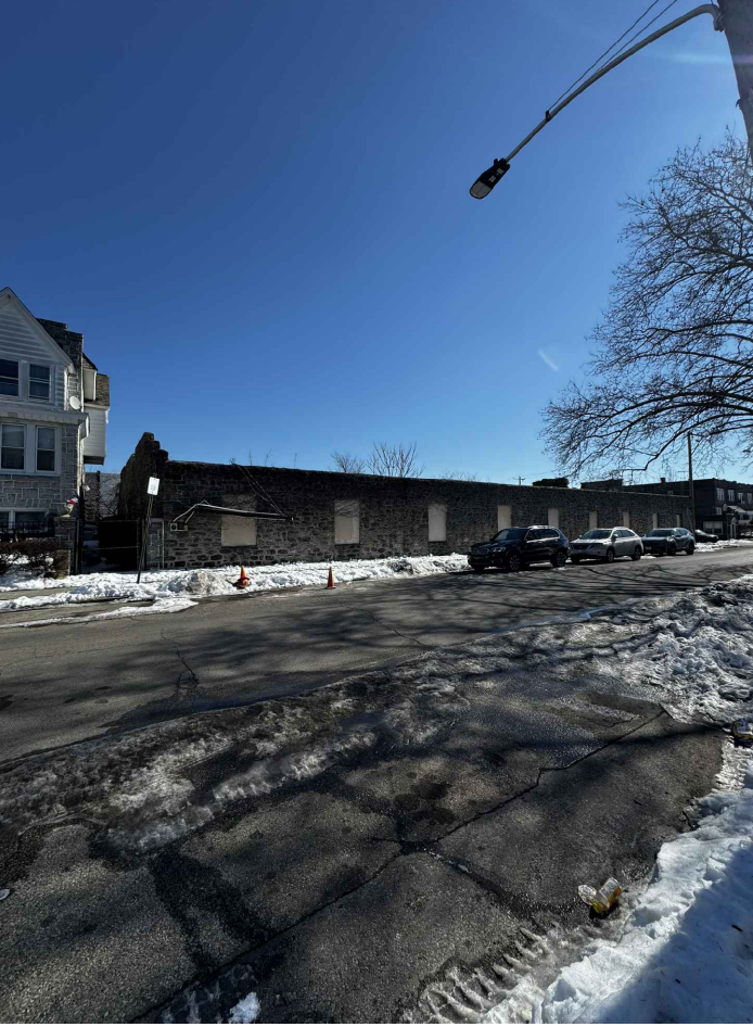
VIEW LOOKING SOUTHEAST - 65TH STREET
