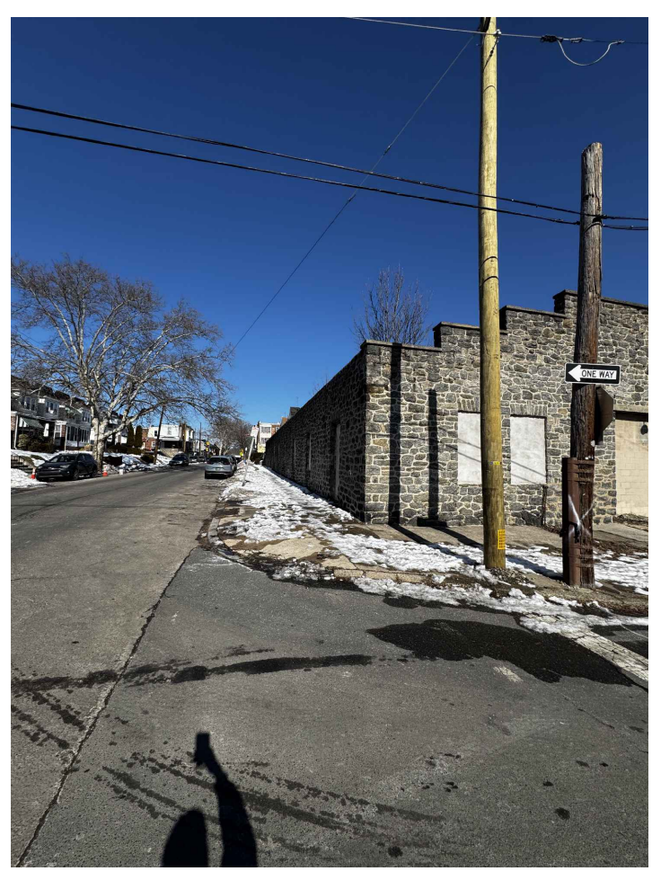
VIEW LOOKING NORTH - 65TH STREET
