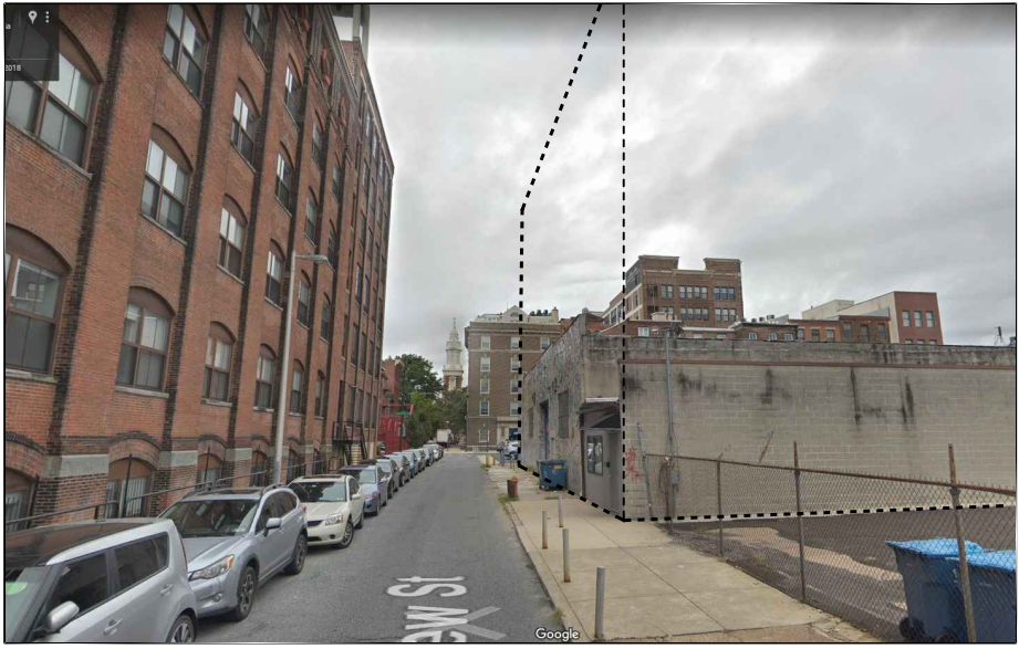
VIEW FROM SE - NEW STREET
