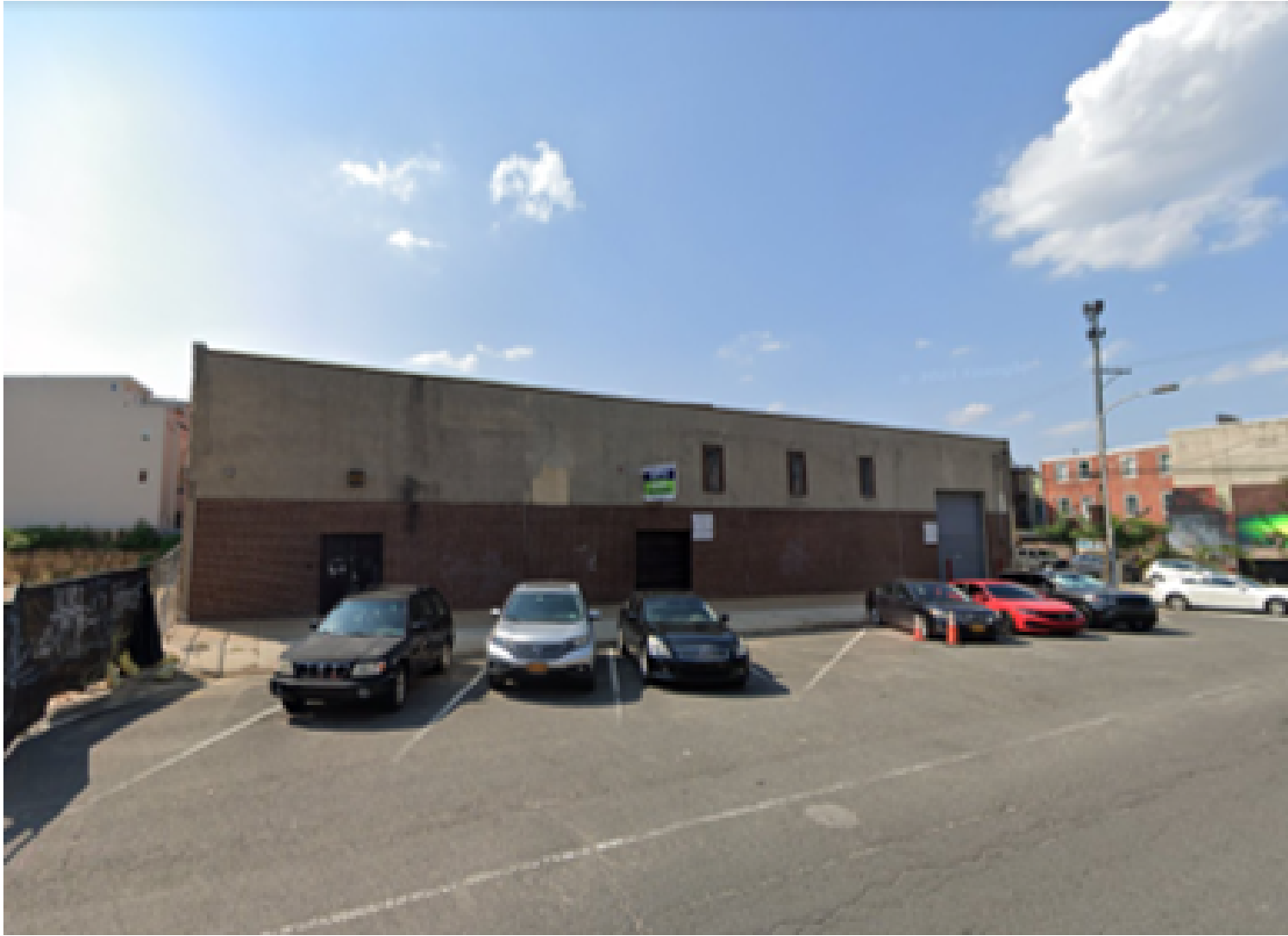
VIEW FROM N. 2ND STREET
