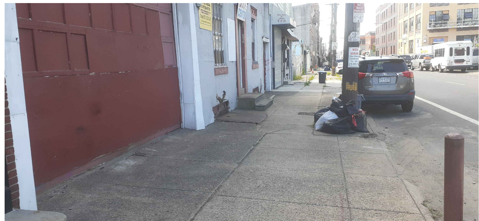
N. 2 ND STREET CURB & SIDEWALK LOOKING SOUTH
