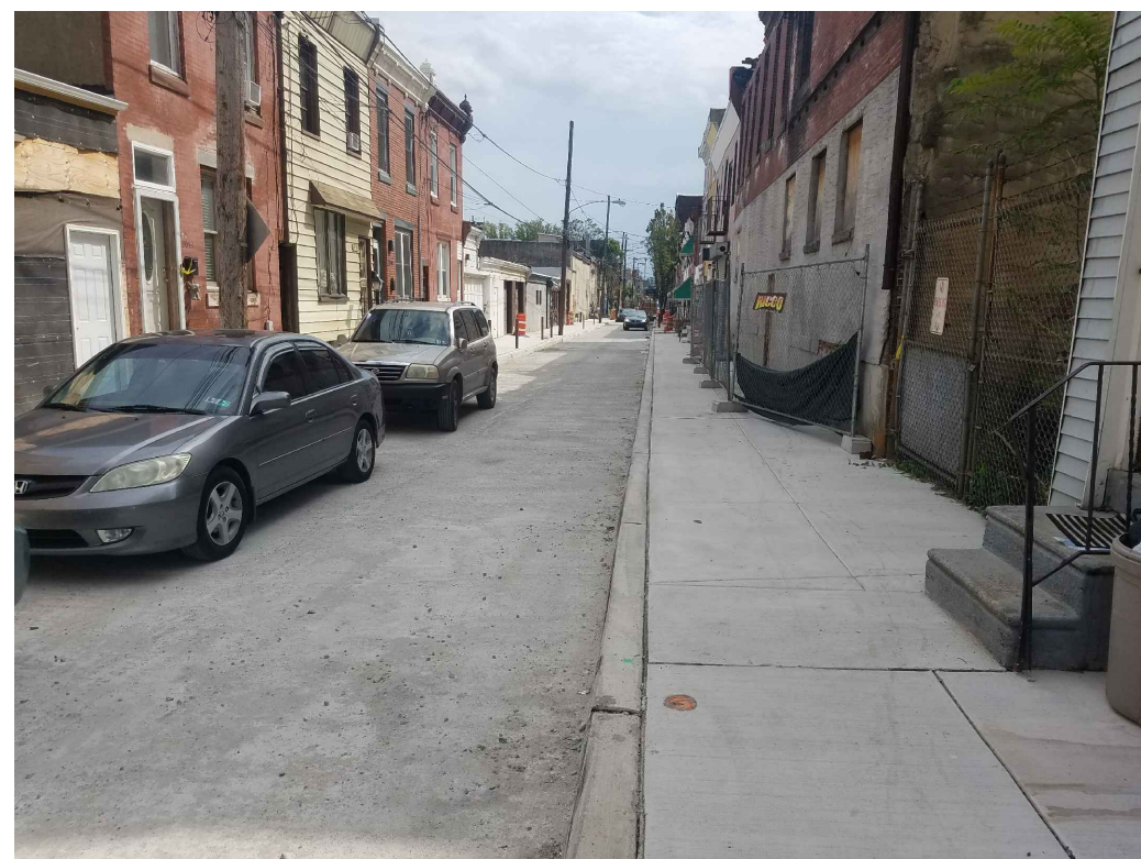
PALETHORP STREET CURB & SIDEWALK LOOKING SOUTH
