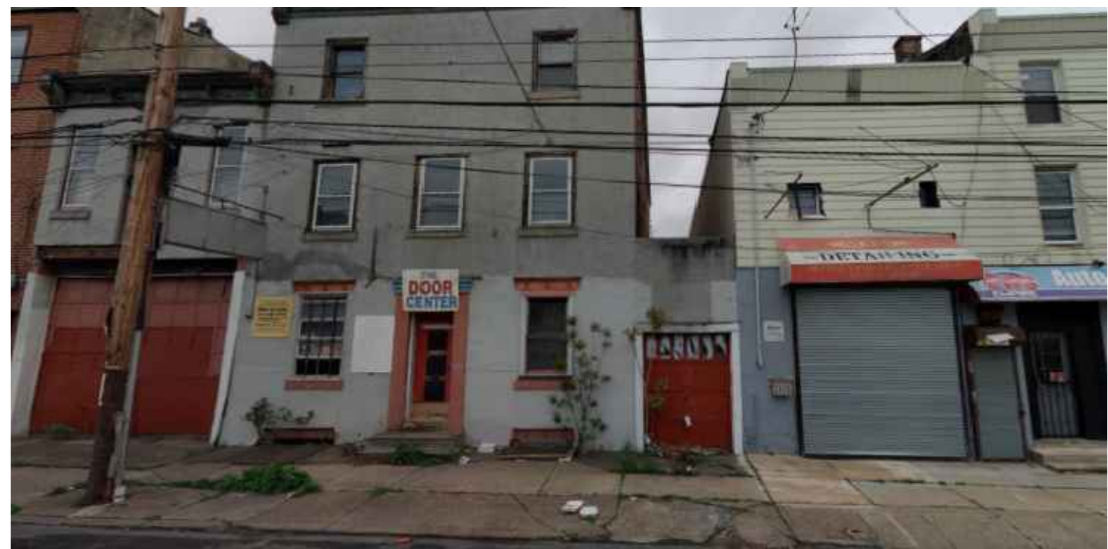
PROJECT SITE LOOKING EAST FROM N. 2 ND STREET
