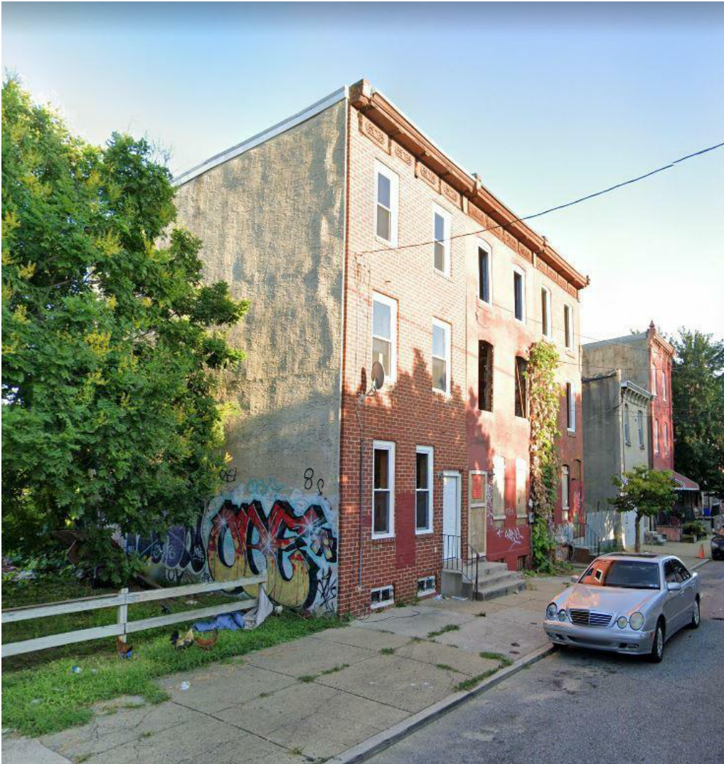
SITE PHOTO: LOOKING SOUTH EAST
