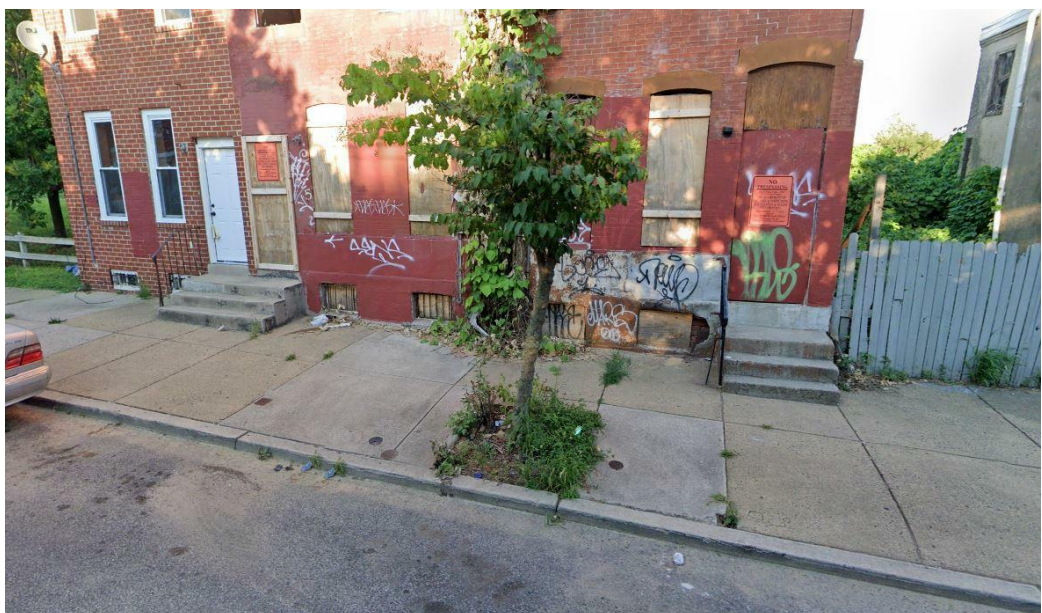
SITE PHOTO: LOOKING EAST
