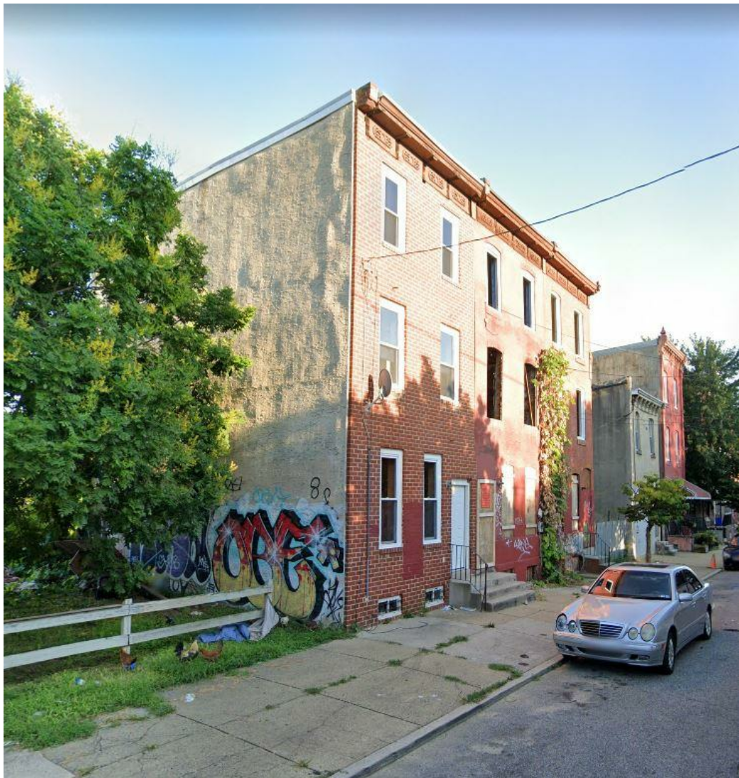
SITE PHOTO: LOOKING SOUTH EAST
