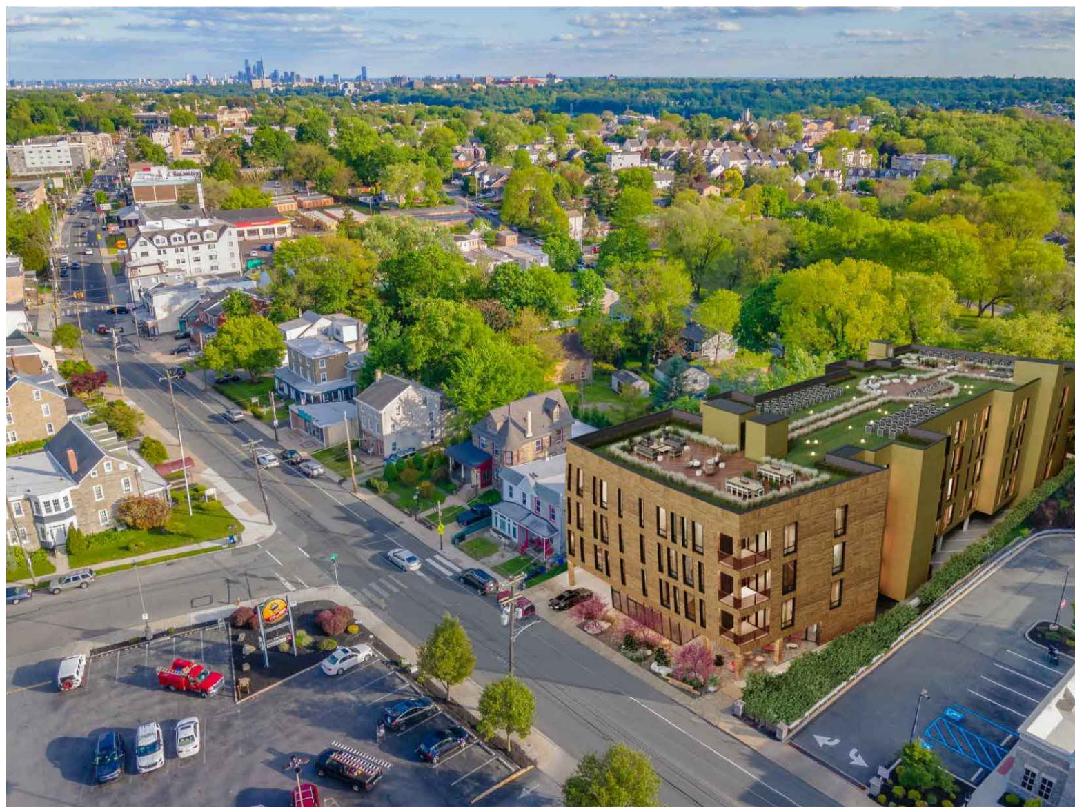
ROOF VIEW FROM NE CORNER NTS
