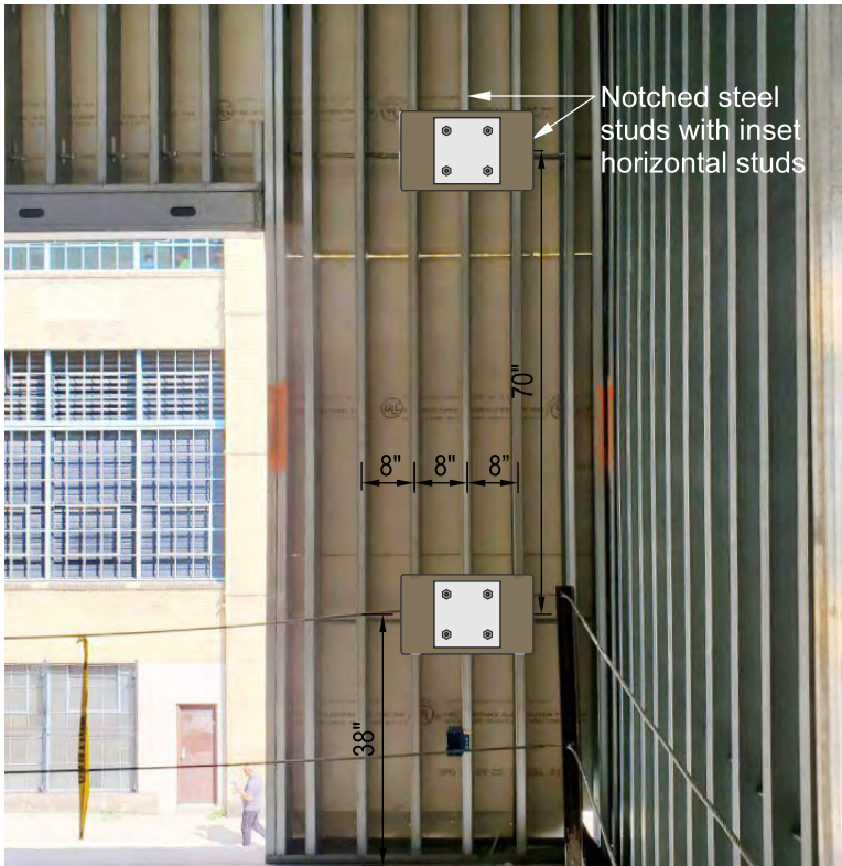
6.0 Interior View - Projecting Sign Blocking Scale: 3/8"=1'-0"
