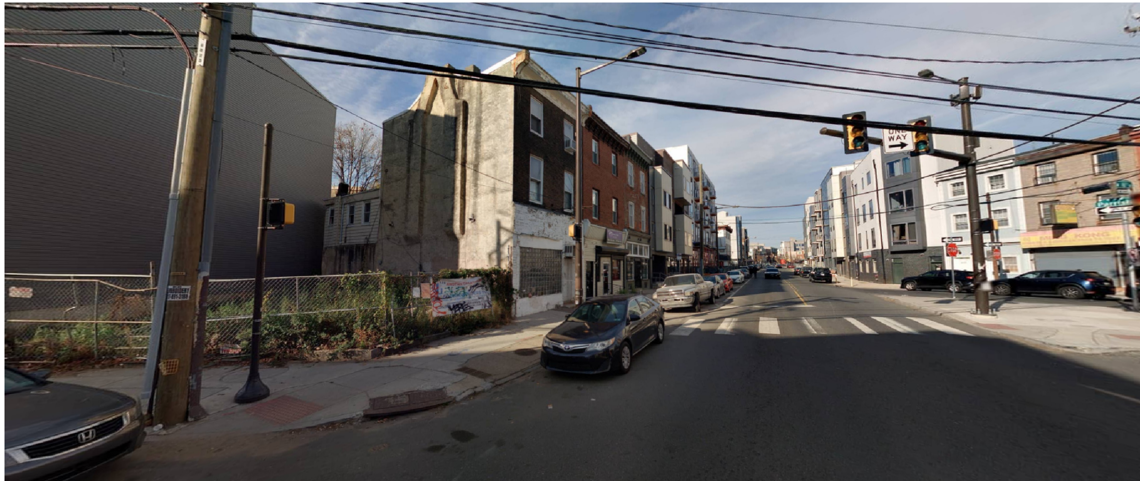
1 PHOTO OF EXISTING CONDITIONS Z-101 / NTS
