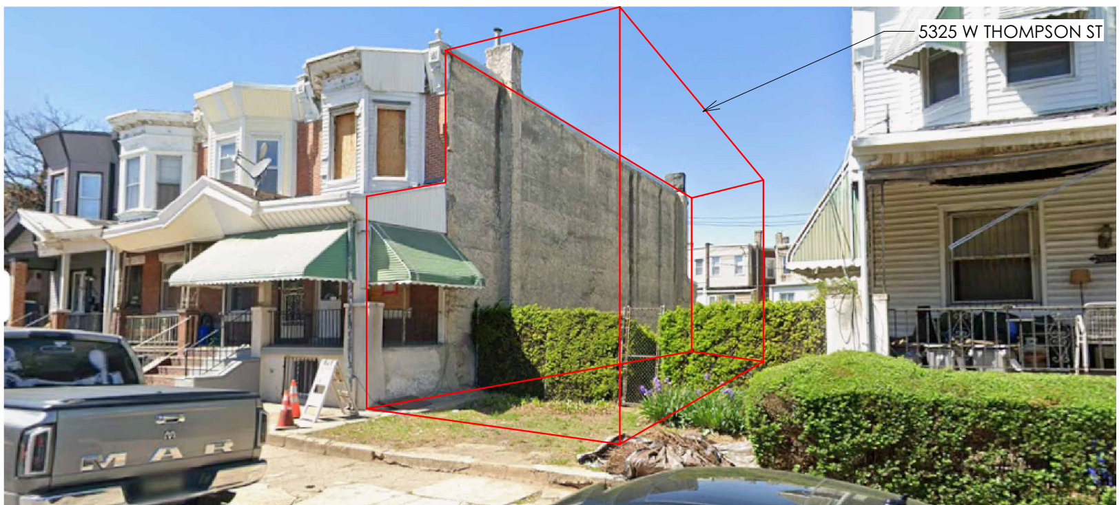
LOOKING NORTH ON THOMPSON ST
